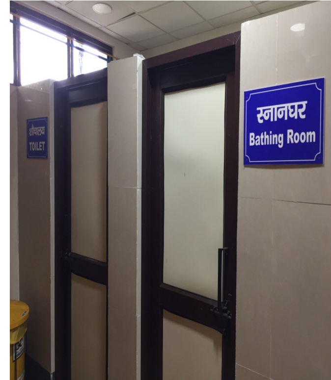
Toilet & Bathing Room
