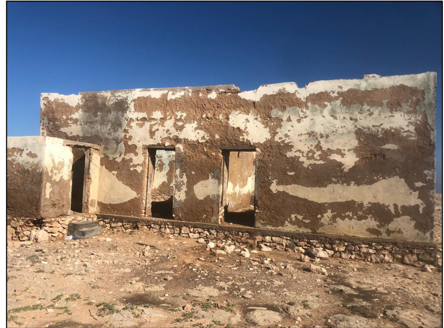
Example of a former HF damaged due to conflict
